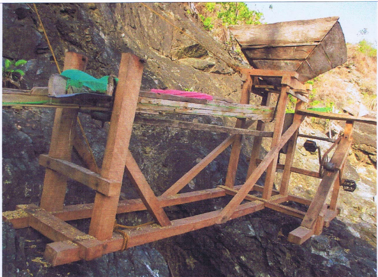
An improvised wooden hopper for screening pebbles into different products sizes, tied up on higher portion on the side of the shoreline when waves are strong. Photo by Rey J. Garcia
